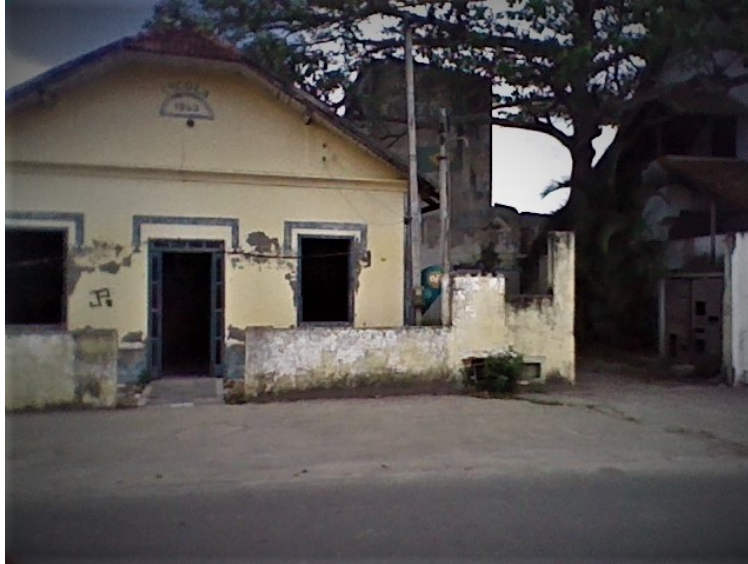
Figure 20- Headquarters of the colony Z-06 in São Pedro da Aldeia
